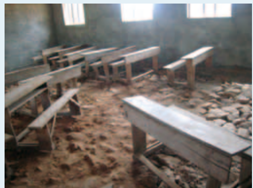
A photo of the partially constructed classroom in Emurutoto primary school
