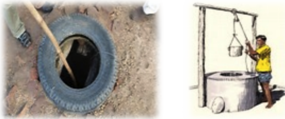
Figure 10.16: Unprotected and protected wells
